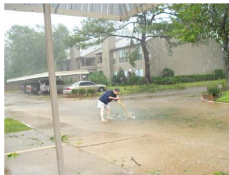
Your Board President checked the property Saturday morning and cleared all the drains to alleviate the worst of the ponding.
