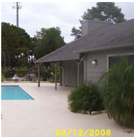
On Friday the clubhouse was all boarded up and ready for Ike.
